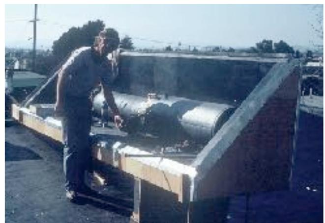
3 Tank Integral Solar Water Heater
