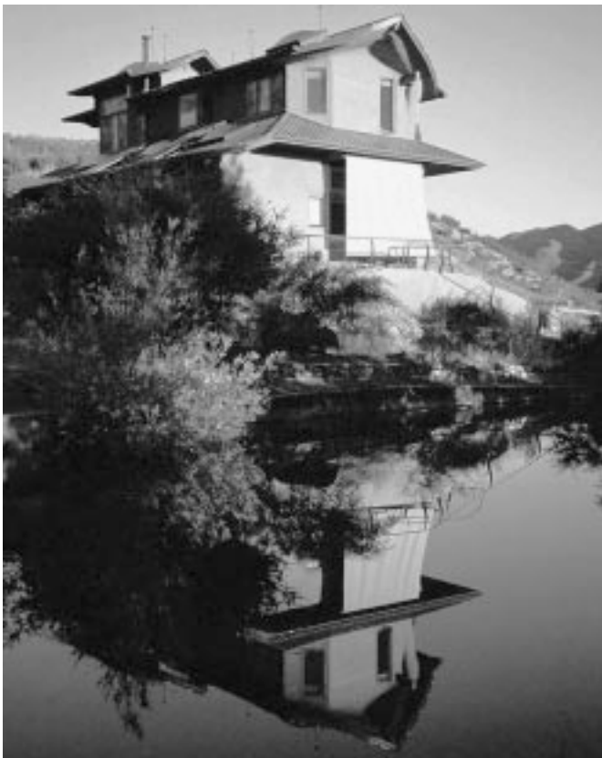
Straw bale seed processing and storage building, San Diego Wild Animal Park, Escondido, Calif., reflects environmental consciousness in more ways than one.
