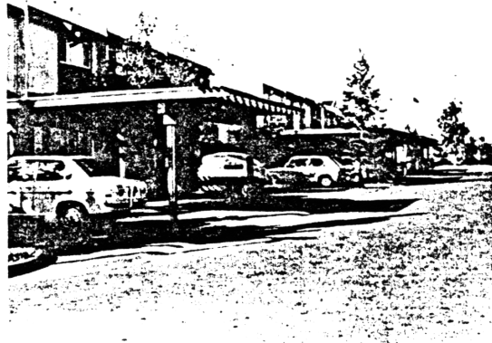
Above: New developments in Davis, California will have narrow streets without street parking. Below: A narrow, tree-shaded street in Davis is one way with two bike lanes and parking.
