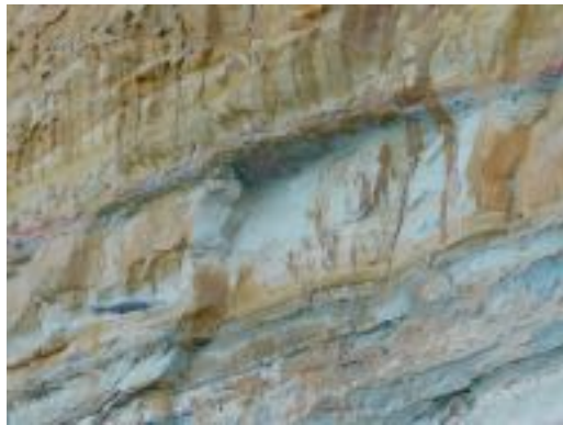
Overhang from recent rock fall, flake to left will go soon - then the cliff face above
