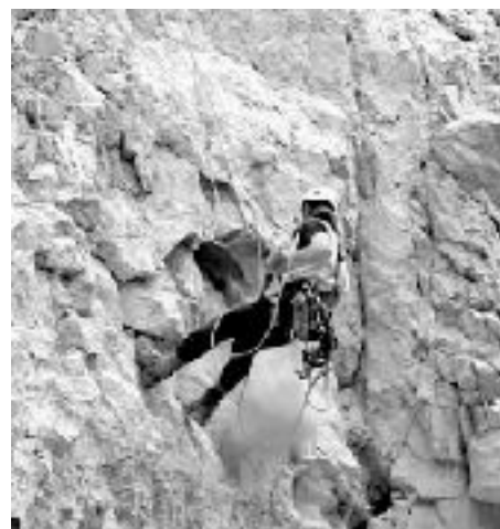
Scaler working on a road cut. Workers become very skilled at this dangerous work. In some cases they haul compressors up the slope to power jackhammers or use dynamite to remove bigger rocks.
