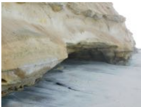
Undercut by waves - eventually will lead to slope failure
