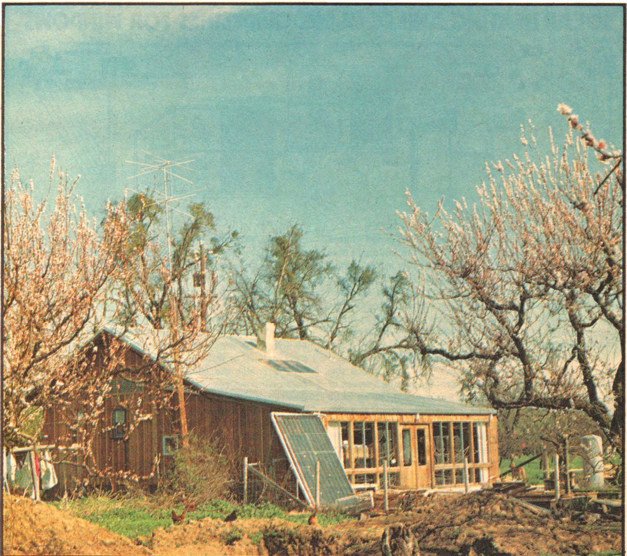
Another view of the Hammond house, showing the solar water heater attached to the home's south wall (in foreground).
